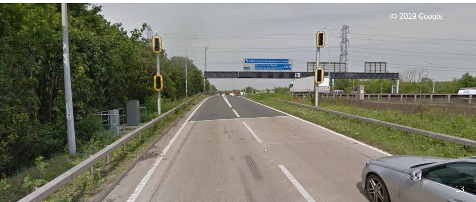
Image 6 – Second generation ramp metering deployed at M25 Junction 13
