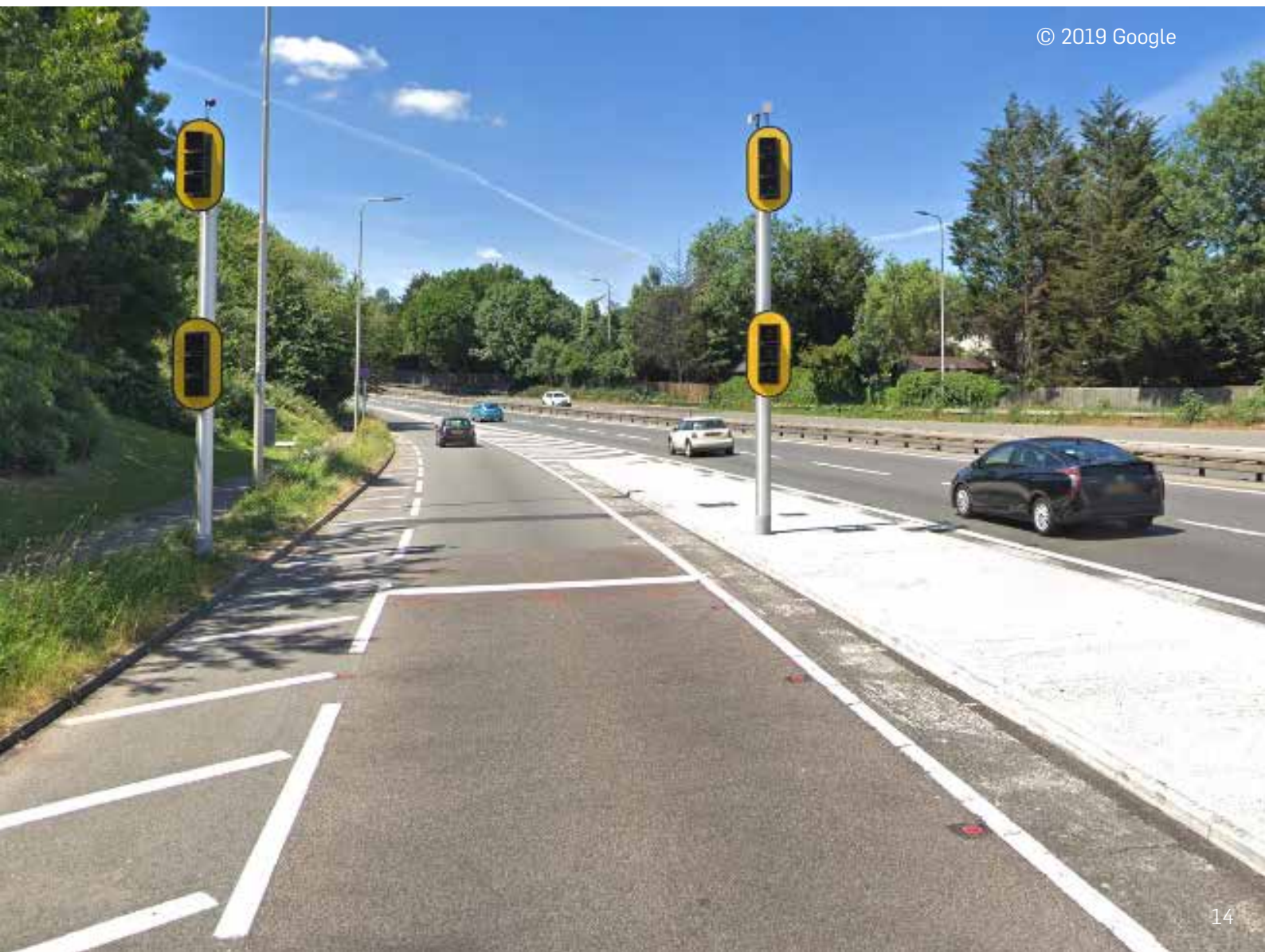
Image 7 - Second generation ramp metering deployed at the A3 in Guildford.
